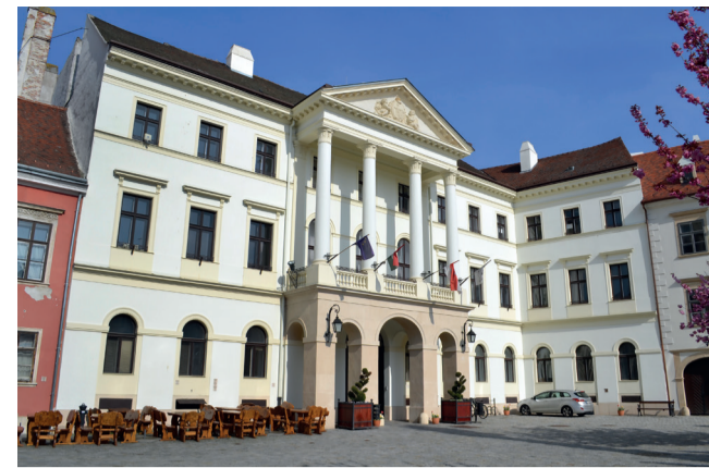
5 The building of the district office (old county hall) in Sopron
