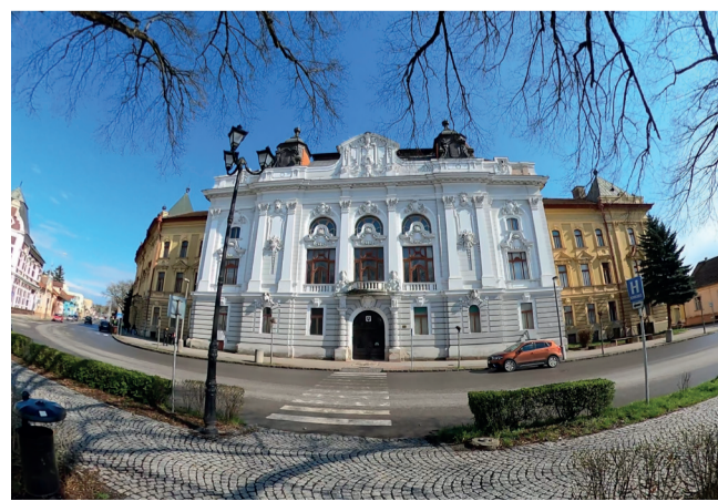
14 District office building in Rimavská Sobota/Rimaszombat
