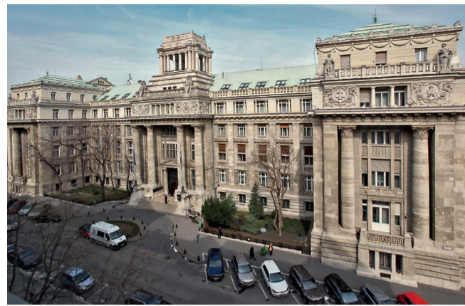
7 The Curia building in Budapest
